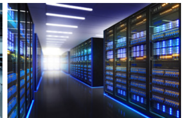
Cooling Distribution Units (CDU)
